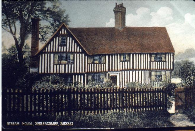
None more so than early 16 th century Durhamford, Stream Lane, here known as Stream House, dated 1913
