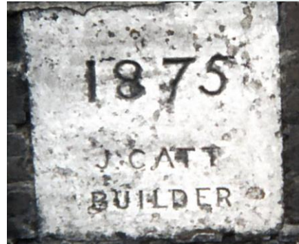
Stone on bridge over River Brede at south of Sedlescombe Village
